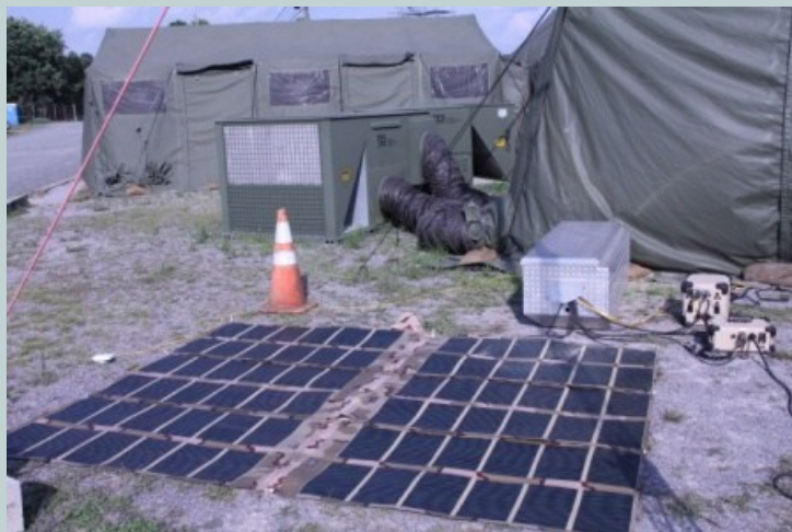
Microgrid systems are currently the only solution that allows the incorporation of multiple technologies, such as renewables and energy storage systems, to supplement traditional power generation techniques. (Photo by Spc. Robert Porter/Released)
