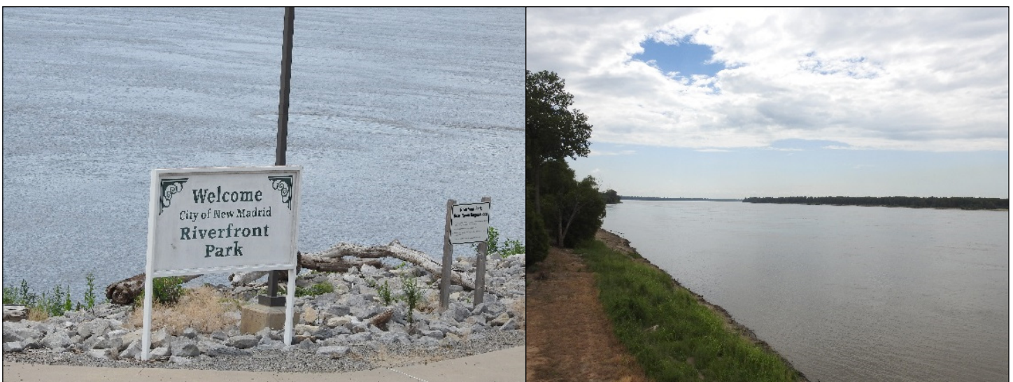
Figure 3: New Madrid's Riverfront Park is sited on top of the New Madrid Levee (right), protecting the town from the Mississippi River. This levee, completed in 1927, is typical of infrastructure that would have to be inspected and possibly reinforced after each significant aftershock. (Photos by author/Released)
