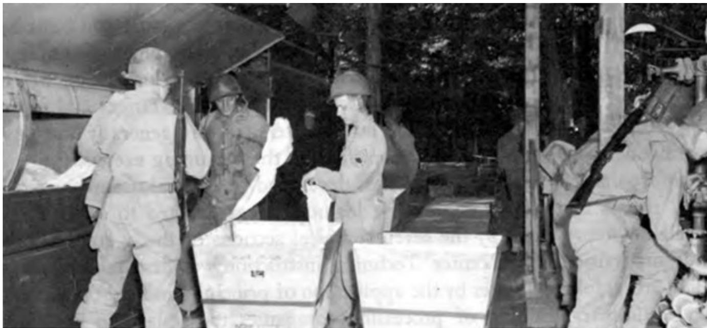
Figure 2-5. Members of a Processing Company in Field Training Remove Clothing From Predryer Unit in the First Stage of the Impregnation Process, and Pipes at Lower Right Carry Gas-Resistant Solution to Impregnator Unit (Source: Brophy and Fisher [38]).
