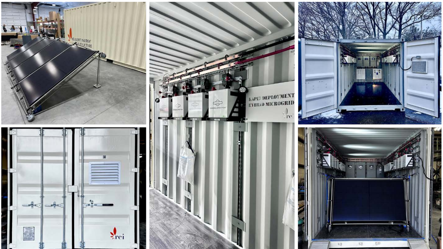
Figure 2. The Built Microgrid With 35-kW ExoSolar, Energy Storage, and Energy Management Systems Integrated Into the Connex (Source: REI).
